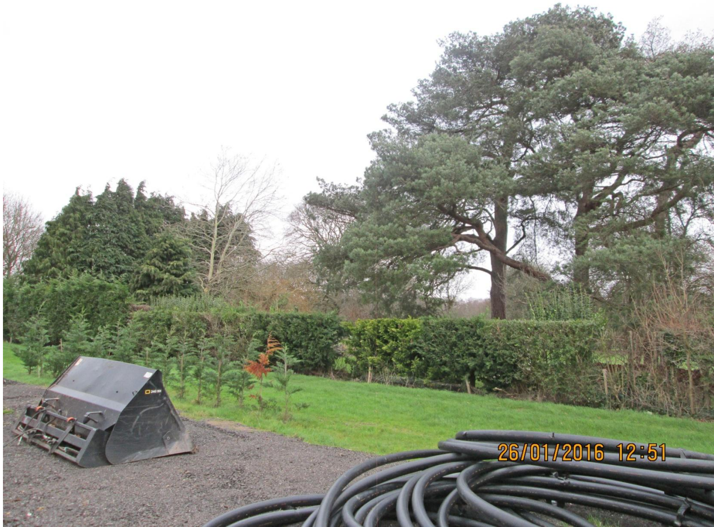
Figure 10 : Eastern Boundary of the Application Site shared with Sutton Ridge House
